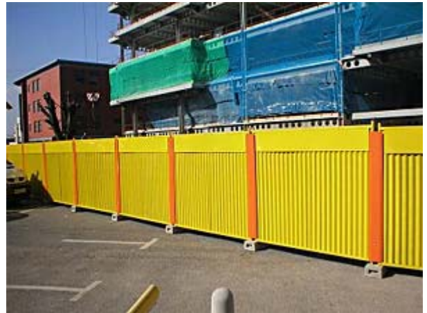
Steel hoarding with infill panels
