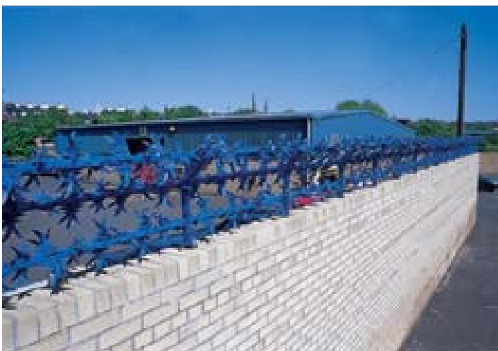
General arrangement of spinner installation.
