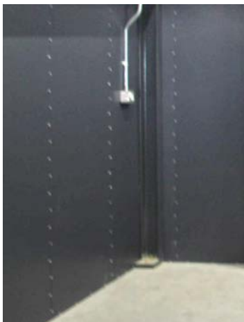
Secure Walling corner detail.
