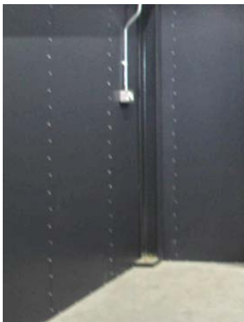
Secure Walling corner detail.
