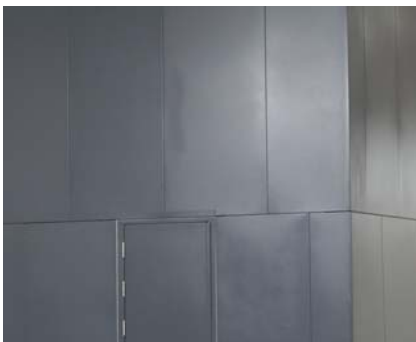
Basic modular panel construction
